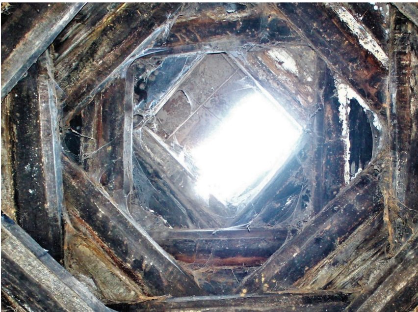
Photograph 41. “Swallow-type” roofing, Baraleti, Meskhetian “Darbazi” (19th-20th centuries)
